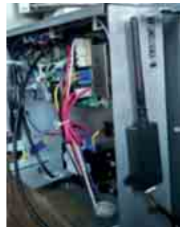
Radio adapter for the indoor unit to be connected to the respective electronic board.
