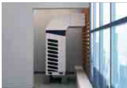
Installation of duct
